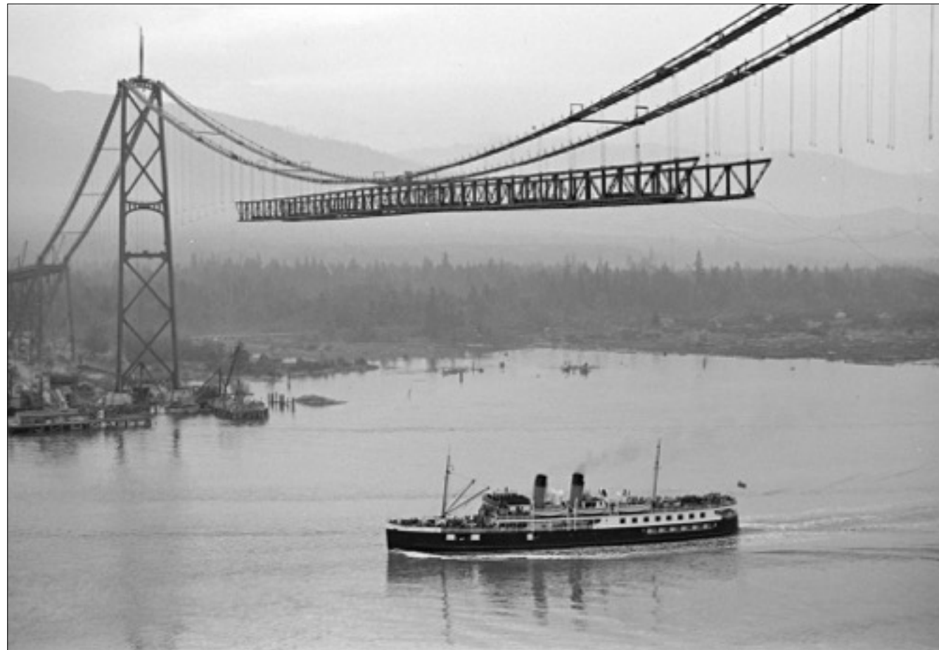
1937 – Lions Gate Bridge construction
